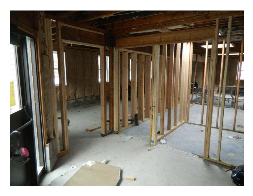
Interior was re-built from the studs (picture taken from entryway)
